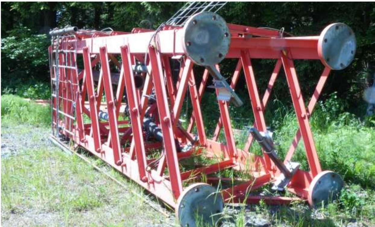
The following picture shows the bottom of the former KUNS-TV Pole. Note the number of large bolts that attached it to the tower.
