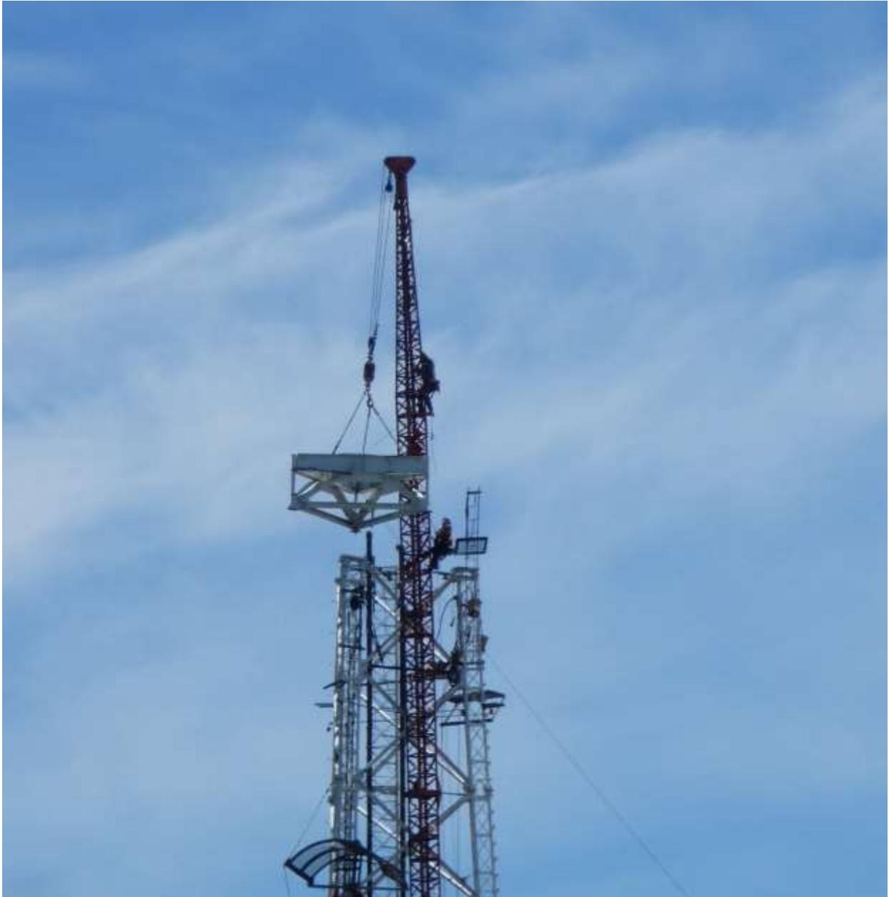
With most of its top pieces now removed, the tower on the right is a lot shorter than the other one. On the other tower, to the left, attached to what's called a 'T-Bar' are two of the site's TV Stations.
