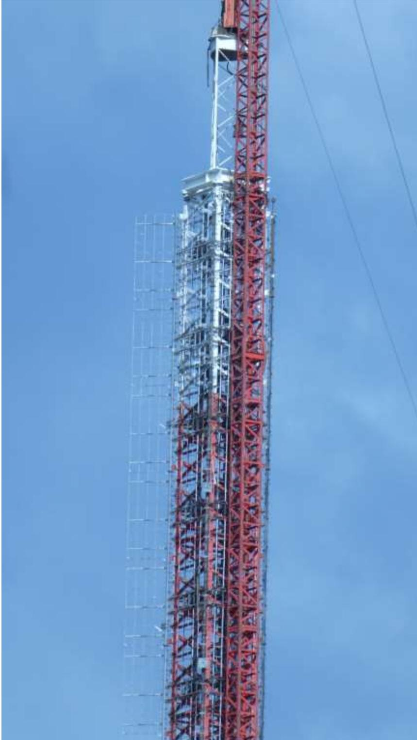
Tilting down some more you can see the rest of the FM's square tower. The big structure painted white is what I call the adaptor that 'adapted' the Triangular tower to the Square one above.
