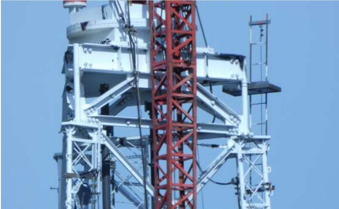
In the following pictures you can see how the Gin-Pole is used to hoist the old adapter off of the tower.
