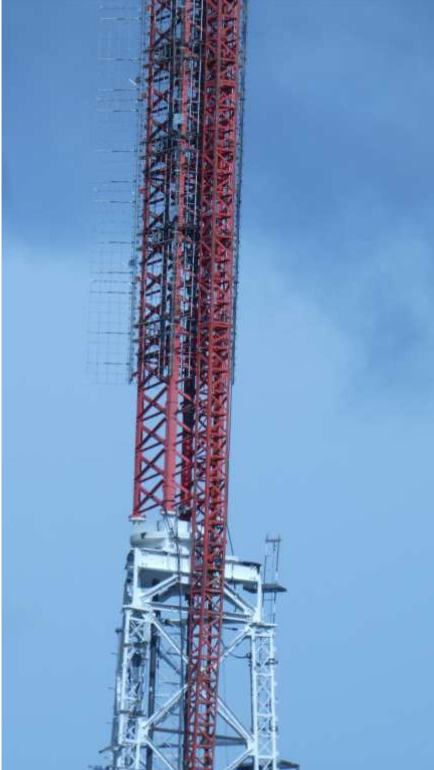
Here's a closeup of the 'adaptor', a very large amount of steel, weighing in excess of 15,000 Pounds. The Red gizmo is the Gin-Pole that has to be strong enough to move these pieces from the ground up here.
