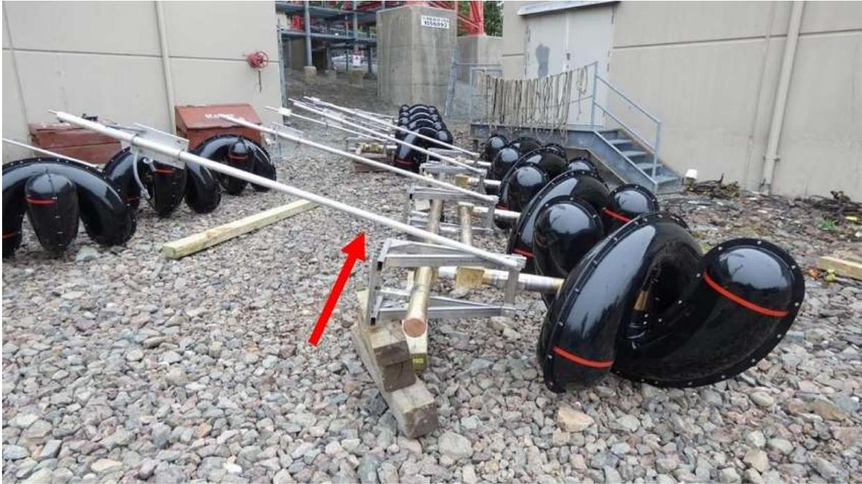
The 16 Antenna 'Bays' or elements are shown here, on the ground. They are all connected together with a lot of 'plumbing', all made of copper and brass.
