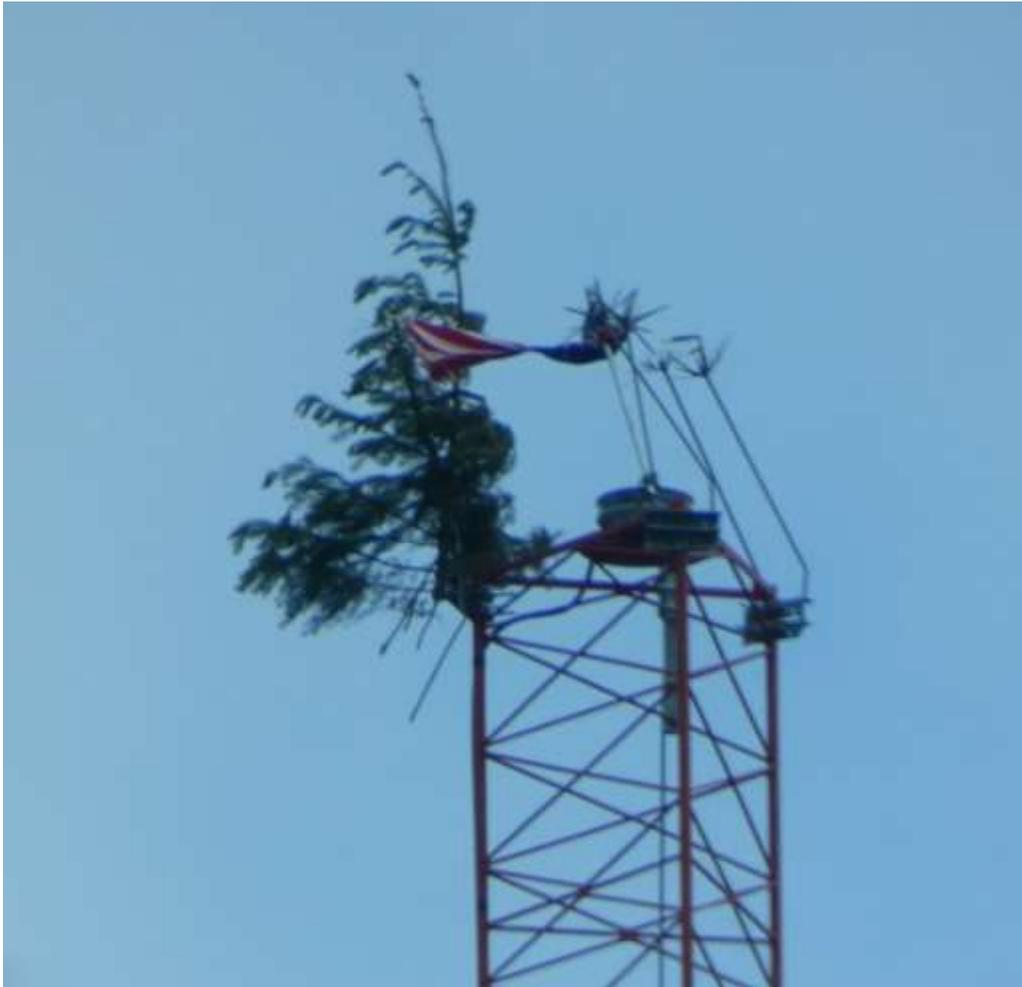
The 'rods' on the left and bent toward the tree are devices designed to deal with lightning. Yes, West Tiger's towers do, indeed, get struck frequently. The round object is the new LED Tower light for the top of the tower. This replaces the old incandescent fixture what was there before. It had not been working for over a year because the wiring was burned in the Antenna Fire.
