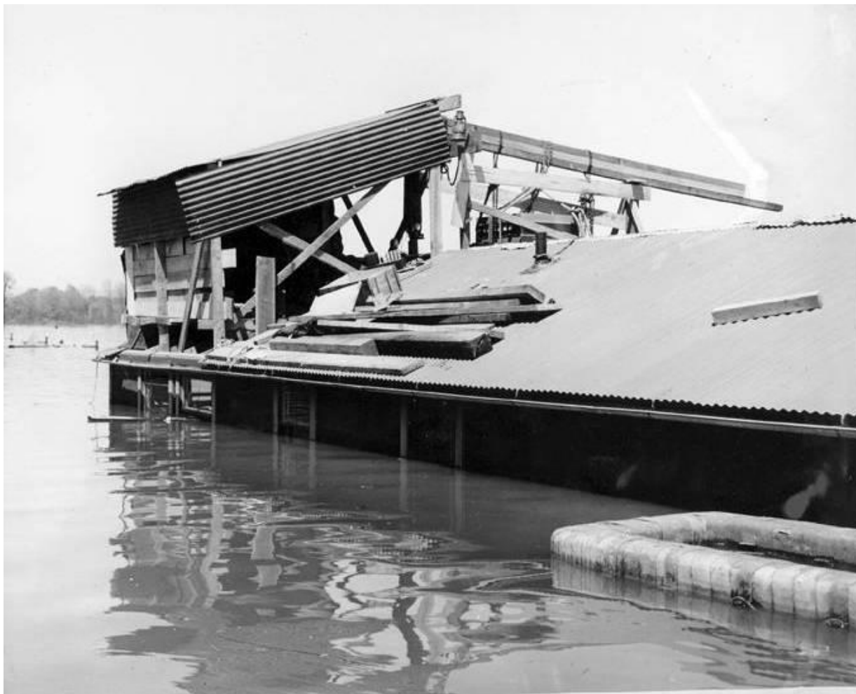
Figure 3-14 The KVAN transmitter building with water up to the eaves. The transmitter protrudes through a hole on the far side of the building, and the makeshift "studio" is perched on the close side. Note the surplus balsa raft in the foreground. (Courtesy Clark County Historical Museum)
