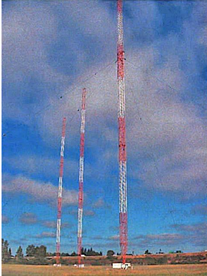
Figure 4-34 Blaw-Knox 455' center-guyed towers erected in 1948. (ODOT 2008)
