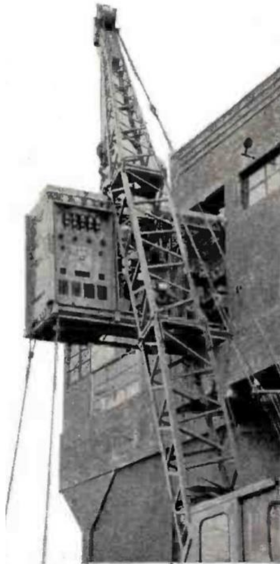
Figure 4-29 Components of the new Raytheon transmitter being hoisted through a third-story window. (Broadcasting 4/11/49)
