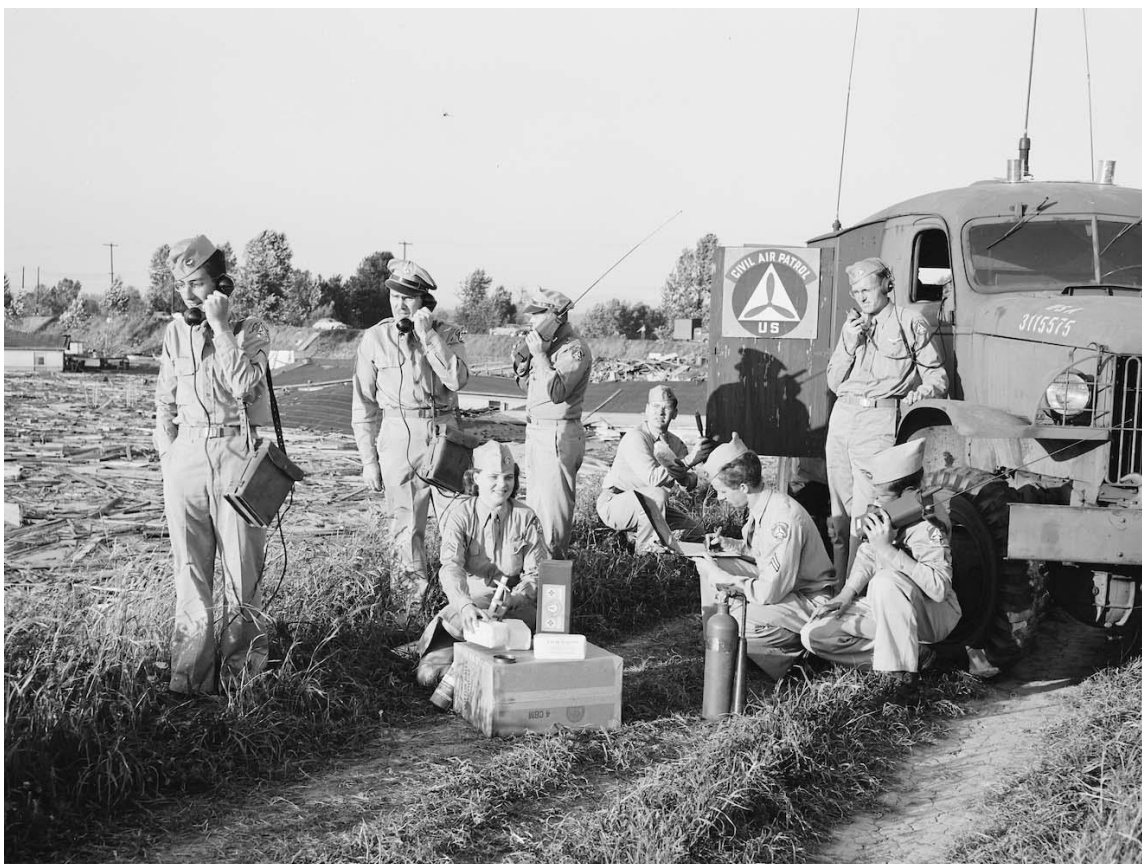
Figure 5-21 Members of the Oregon CAP pose with their heavy radio truck, a 1941 Chevrolet 1-1/2 ton panel truck. Antennas dot the roof. CAP members are demonstrating EE-8 field telephones and BC-611 Handie-Talkies. Staff Sgt Ethyle Kremers is seated behind the desk. (Akroyd photo) (Courtesy Historic Photo Archive)
