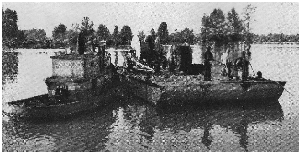
Figure 5-37 Laying emergency cables by-barge. (Pacific Telephone Magazine)
