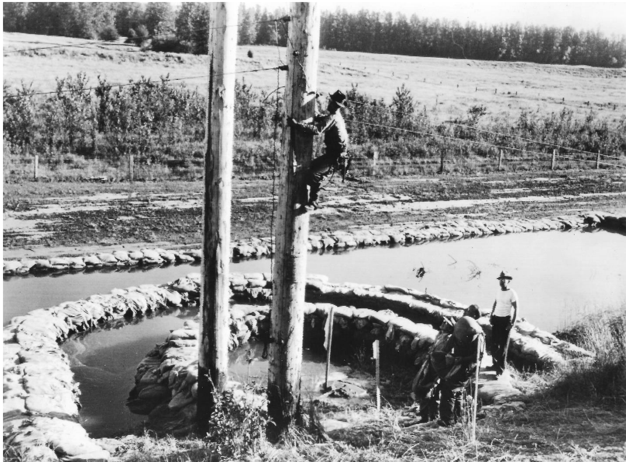
Figure 5-32 Utility workers install temporary lights for keeping tabs on the dike near Troutdale. Three rings of sandbags help stop a "sand boil" on the dike's edge from turning into a breach. (The Oregon Journal 6/6/48) (ACME Telephoto)
