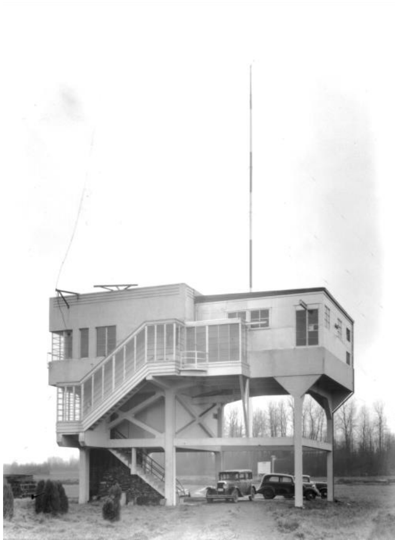
Figure 4-23 East view of the KGW transmitter building in 1934 with the KEX wooden mast in the background. Note that the top floor has been significantly expanded. The lower portion of the building was enclosed in 1949 when the facility was rebuilt. This created a ground-floor garage space and an apartment on the second floor.
