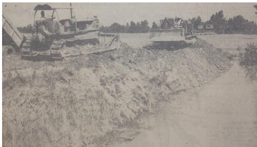
Figure 6-8 Repairing the Union Avenue fill. (The Oregonian)
