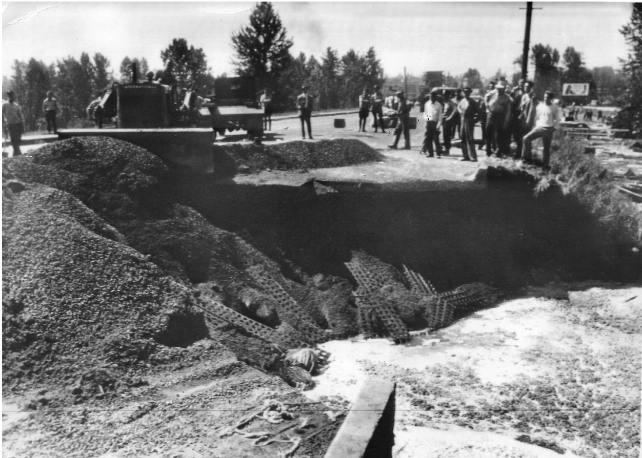
Figure 6-2 Water boils against the Vanport-side of the Denver Avenue fill at the site of a failed culvert. Workers are using a bulldozer to push rock and surplus aircraft landing strip mats into the gap in an effort to prevent a breach. (ACME Telephoto)
