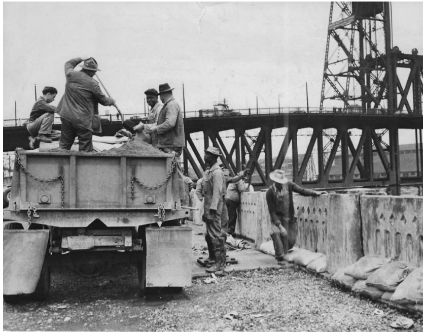
Figure 3-2 A City of Portland crew sandbags the seawall just upstream from the Steel bridge. Erected in 1912, the Steel Bridge is the only double-deck bridge with independent lifts in the world. In this view, water has almost reached the lower (railroad) deck. The upper deck, carrying automobiles and electric streetcars, is well beyond the reach of the water.
