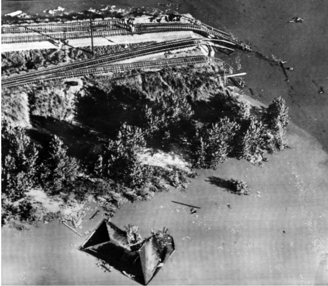
Figure 4-3 Breached railroad fill photographed on Monday May 31 st , 1948. (ACME Telephoto.)
