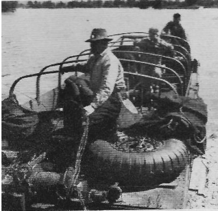
Figure 5-36 Senior Repairman Vic Turnbull crouches in the stern of an army DUKW "Duck" as duplex telephone wire is pulled across the Denver Avenue gap. (Pacific Telephone Magazine)
