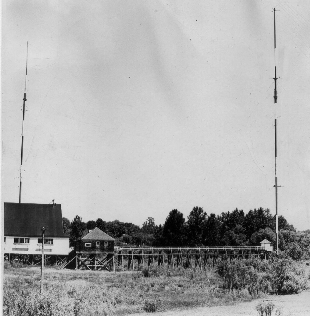
Figure 3-19 KWJJ transmitter building and towers at Oaks Park ca. 1940. Note the trestles carrying the transmission lines out to the towers.
