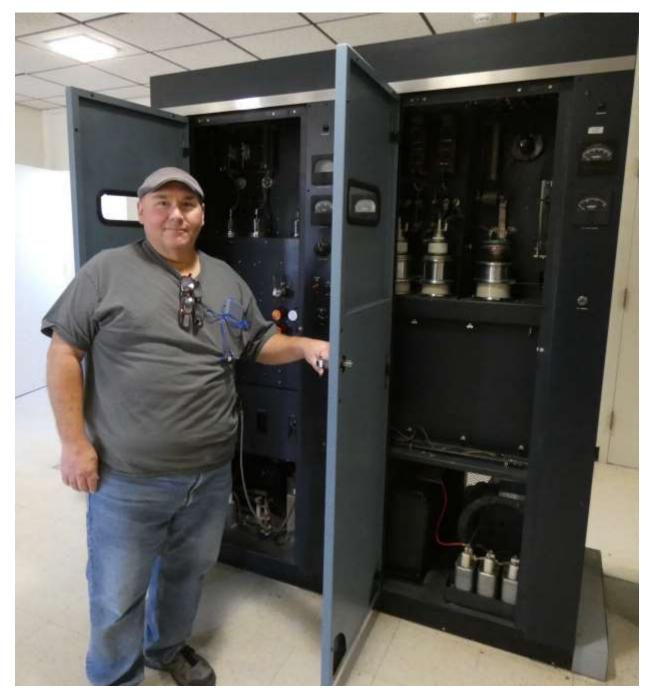
Here's a picture of NWPB Engineer Jim Boothby standing in front of that RCA, with the doors open. Yes, this was a Vacuum Tube Transmitter. Made before solid state transmitters were thought of.
